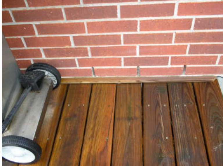
Cracks in garage concrete observed, typical.
