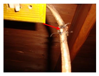
Electrical conduit is not secured to base of condensing unit disconnect.
