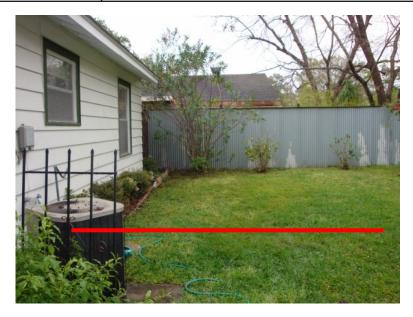
Soil level too high around areas with wood siding. Code and common industry practice requires a clearance of 6-8 inches from bottom of wood veneer to soil. High soil level near wood siding promotes water/termite penetration and wood rot.
