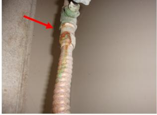
Located in house without benefit of a drain pan. Should water heater leak interior flooring can be damaged REF.: 1991 Standard Plumbing Code 1213.7.1 IRC 2801.5.
